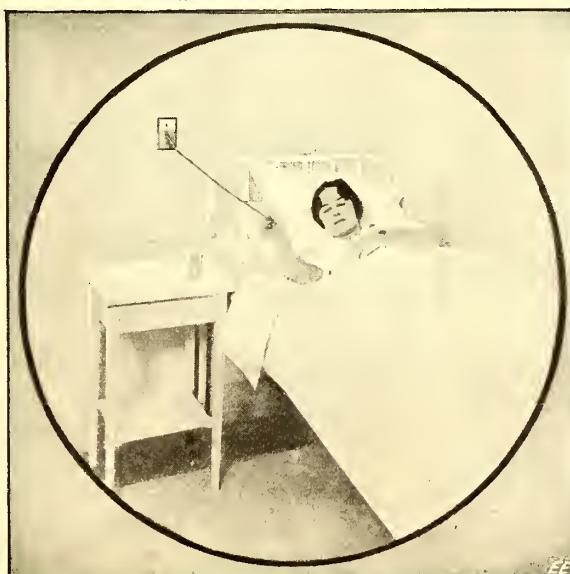
A New Hospital Call Switch. Individual Indication At Each Bed Is Effected. The Nurse Cannot Ignore It.
